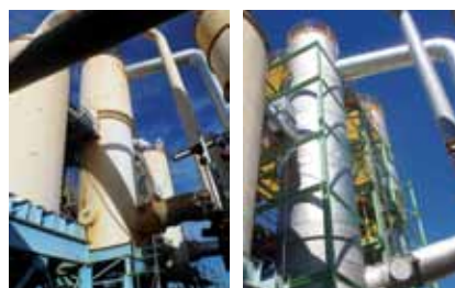
Before: the ducting was suffering from corrosion. After: replacements will mean more reliable operation and less risk of leaks.
