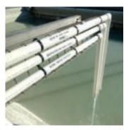
The internal piping system minimises leaks, syphonic pumps pull large water volumes from the roof and the pond allows water recycling in the manufacturing process.
