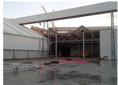
Christchurch Works new intake (with old intake in the background)
