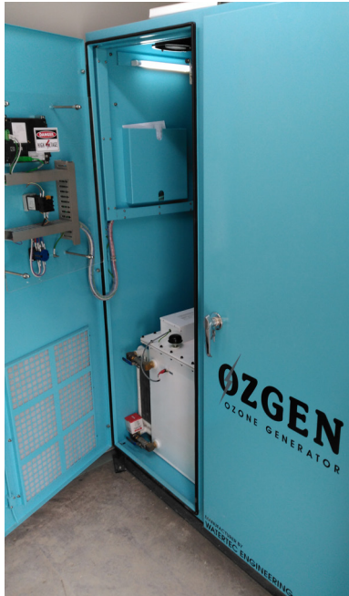
Dunedin Works new ozone generation and injection unit
