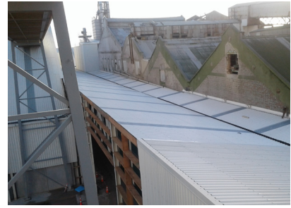
Christchurch Works new central alleyway
