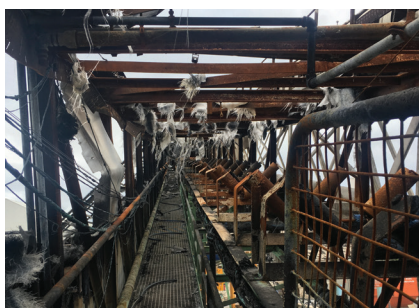
Before and after: the fire seems to have started in the conveyor intake system.
