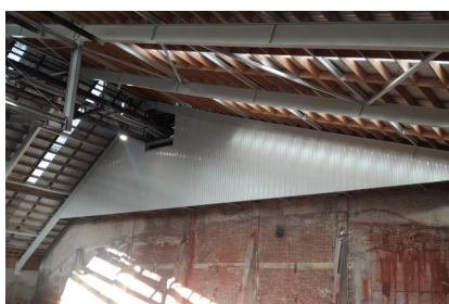
Before and after: the roof and cladding in store 15 was completely replaced before taking delivery of a potassium chloride shipment.
