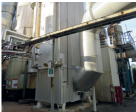
Christchurch and Dunedin Acid plant Economisers: Replacement of end-of-life asset to increase reliability, lower repairs and maintenance costs.
