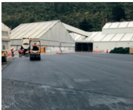
Dunedin Works' yard sealed surfacing improved environmental performance and reduced nutrients in stormwater.
