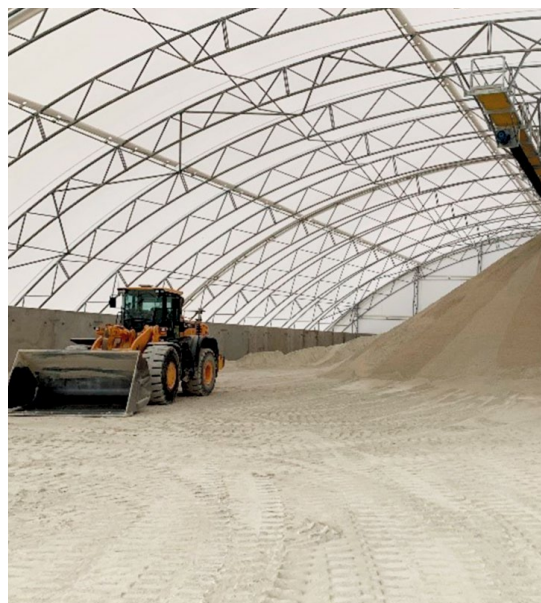
New lime shed at Supreme Lime to increase availability and operational efficiency.
