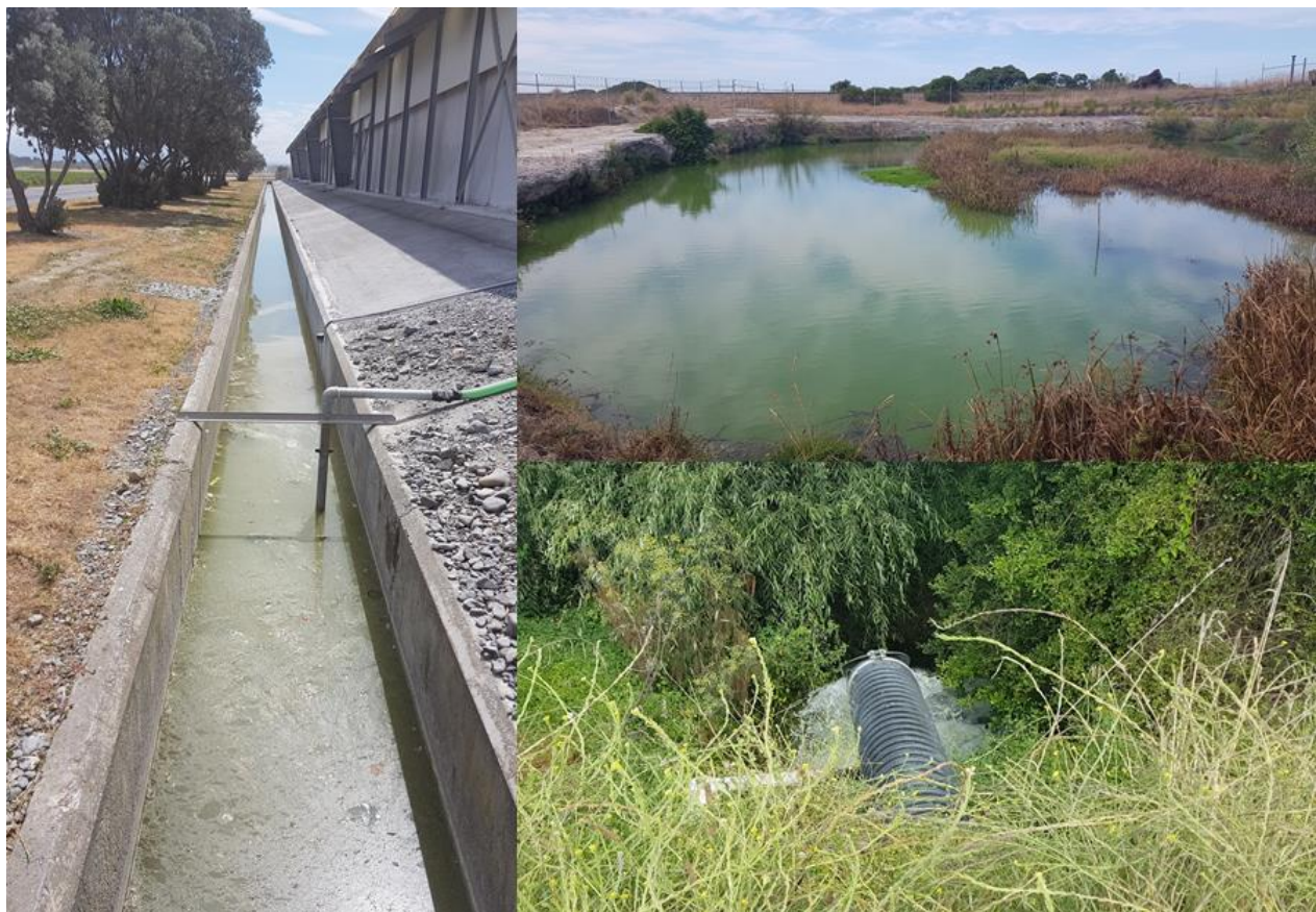
Figure 1. Stormwater drain adjacent to the Ravensdown facility (left), settling pond (upper right) and discharge pipe to Ravensdown Drain (lower right).
