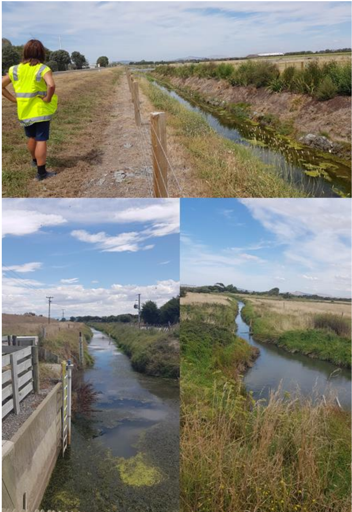
Figure 3. Waitangi Drain upstream/adjacent to the Ravensdown facility (upper), confluence of Mission Drain and Awatoto Drain with HBRC pump station and stop bank visible (lower left) and Awatoto Drain downstream of the stop bank (lower right).
