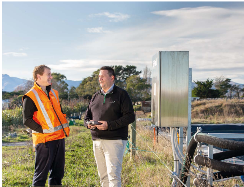
EcoPond treats dairy shed effluent by adding iron sulphate to an effluent pond.
