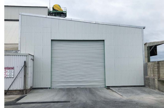
Severn Street Store in Napier despatch before (top) and after (bottom).
